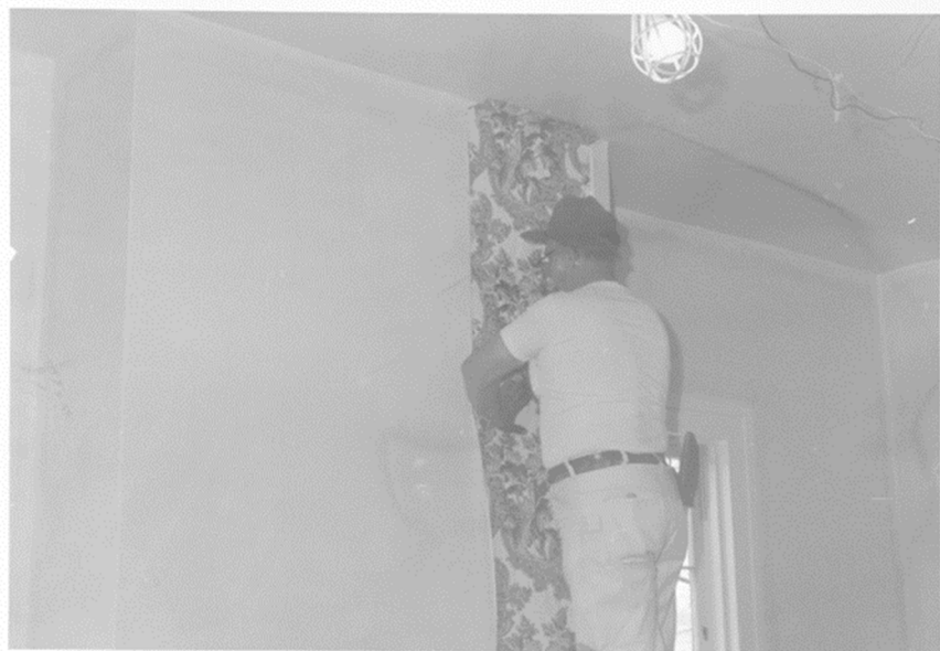
Figure 5: (Left) Restoration of Mary Lincoln's Bedroom. Man pasting reproduction wallpaper. Ca. 1988. Photograph by Joe Winkleman, National Park Service.
