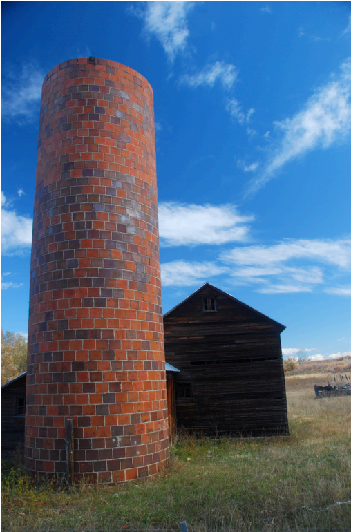
Figure 5: Fired clay tile silo located near Boulder, Colorado.
