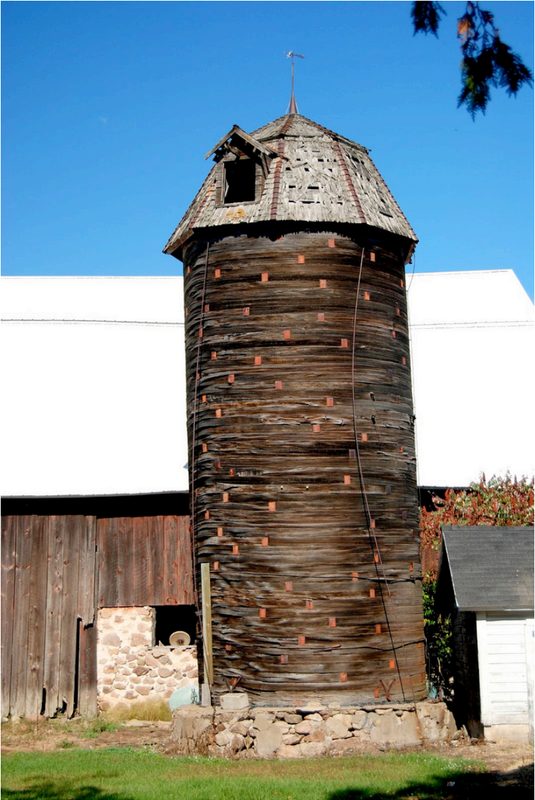
Figure 3: Wooden hoop silo near Gresham, Wisconsin. Note the dormer on the roof.
