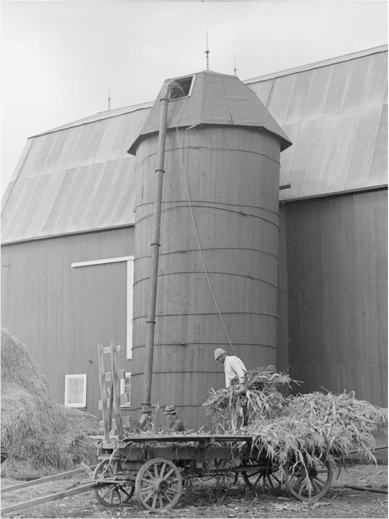
Figure 2: Wooden stave silo in Tompkins County, New York, September 1937. Source: Library of Congress, U.S. Farm Security Administration, Office of War Information.
