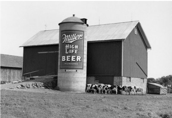
Figure 8: A slip-form concrete silo located near Madison, Wisconsin. Photo taken July, 1937.
