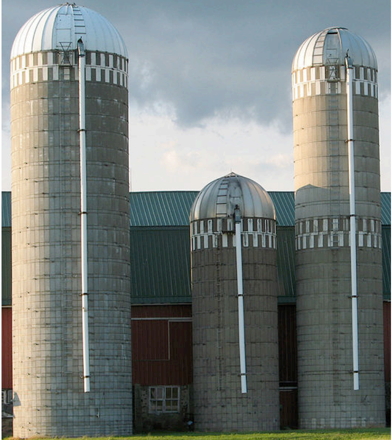
Figure 6: Concrete stave silos of varying height and diameter. These silos are built with automatic unloaders, seen by the use of small diameter chutes on the side of the structure. This type of silo is still built today. Location unknown.
