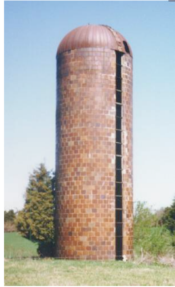
Figure 10: Fired clay tile silo. Note the continuous door slit, which is bridged by reinforcing rods. There is also no visible ladder, so in this case the rods may have served a dual purpose as a ladder as well. Located near Ashburn, Virginia.
