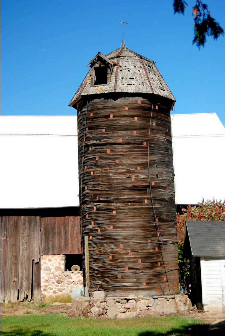
Figure 3: Wooden hoop silo near Gresham, Wisconsin. Note the dormer on the roof.
